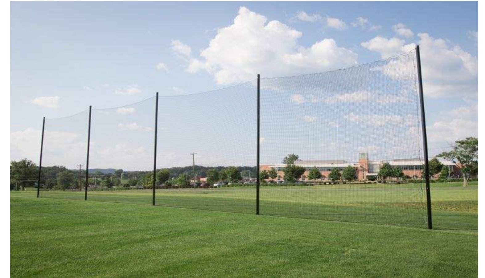
Semi-Permanent (sleeved) Netting for Soccer 20' height
